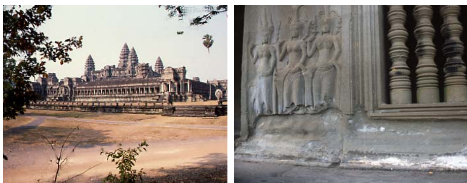
Fig. 1a, b: General view of the Angkor Wat temple from southeast (a, left) and detail with contour scaling of the sandstone and salt efflorescence in a gallery (b)
