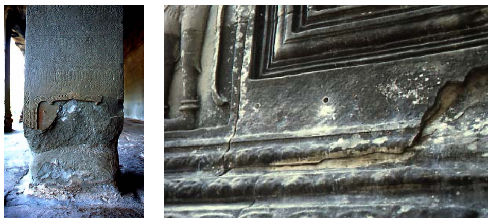
Fig. 4 a, b: Pillar from the northern gallery of the third enclosure (a, left) and surface with contour scaling (b, right)
